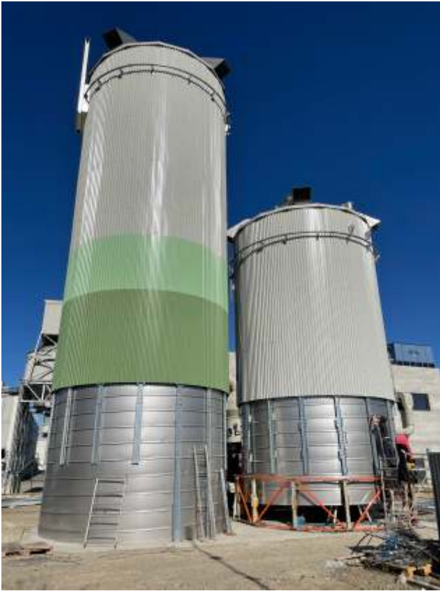
Stainless steel smooth spiral silos having flat bottom and individually insulated.
