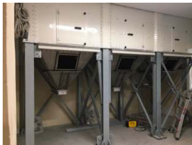
Flat wall cells battery, smooth sandwich-type, for conditioned wheat storage, on a metal structure.
