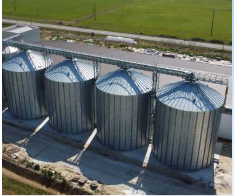
Flat bottom corrugated bolted silos.
