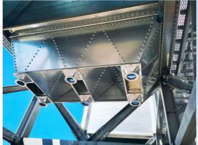
Flat wall cells battery with multiple discharge hopper for blended product/conditioned wheat storage.
