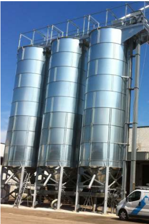
Smooth bolted silos on single pillars.
