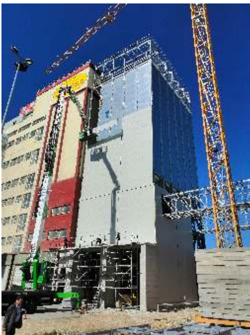
Flat wall cells battery, smooth sandwich-type, on a metal structure for bulk semolina trucks load.
